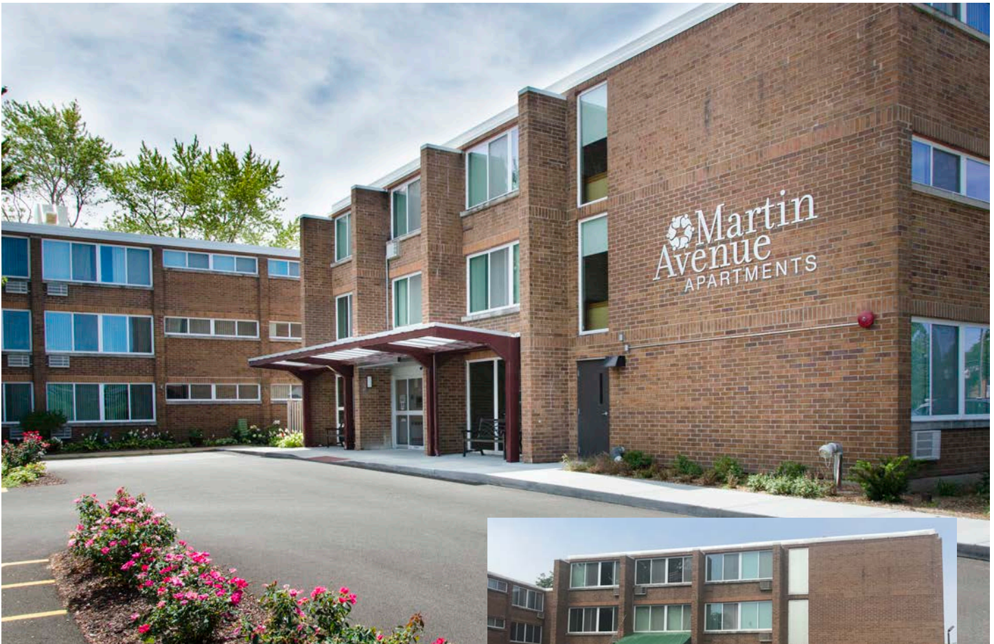
Entry after renovation
